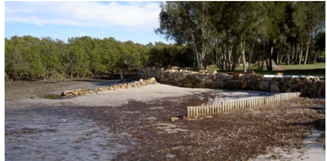
(2) Strewn rock rubble, tyre, rock and pole groyne foreshore protection structures.
