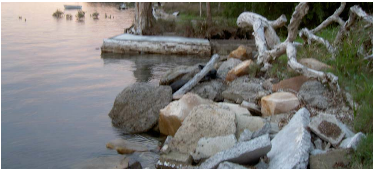
(2) Concrete rubble revetment.
