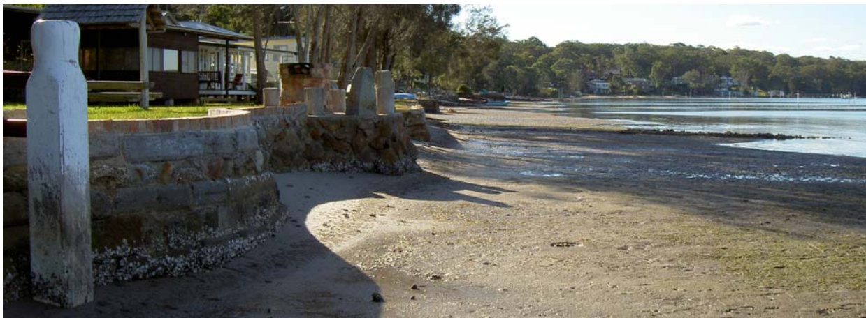
(2) Foreshore reclamation and grouted vertical masonry sea wall – south end.
