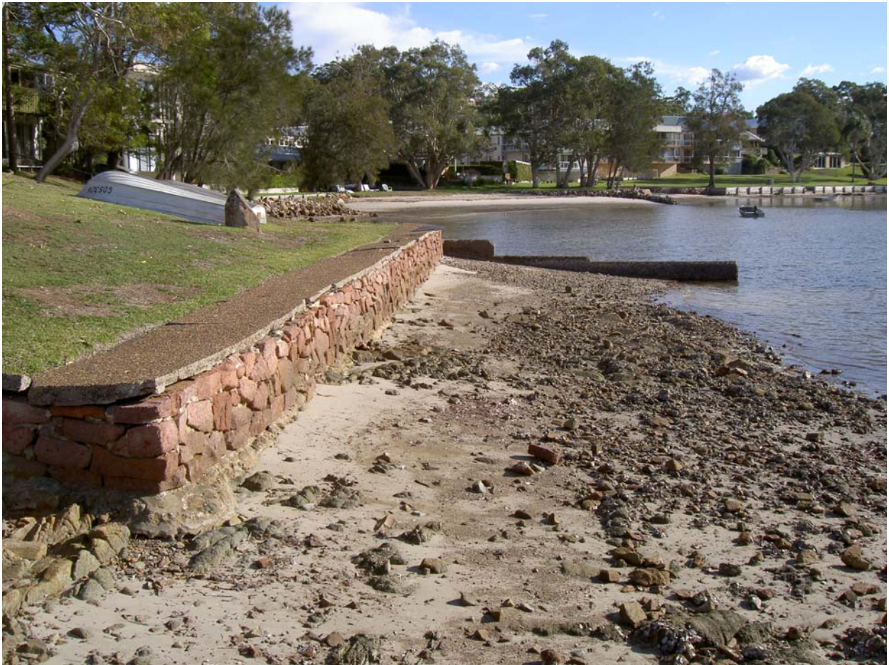
(1) A range of seawalls and groynes along this foreshore
