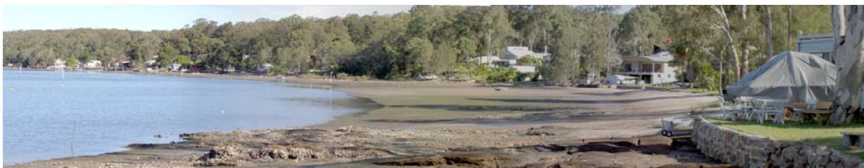
(1) Foreshore reclamation and grouted vertical masonry sea wall – north end.
