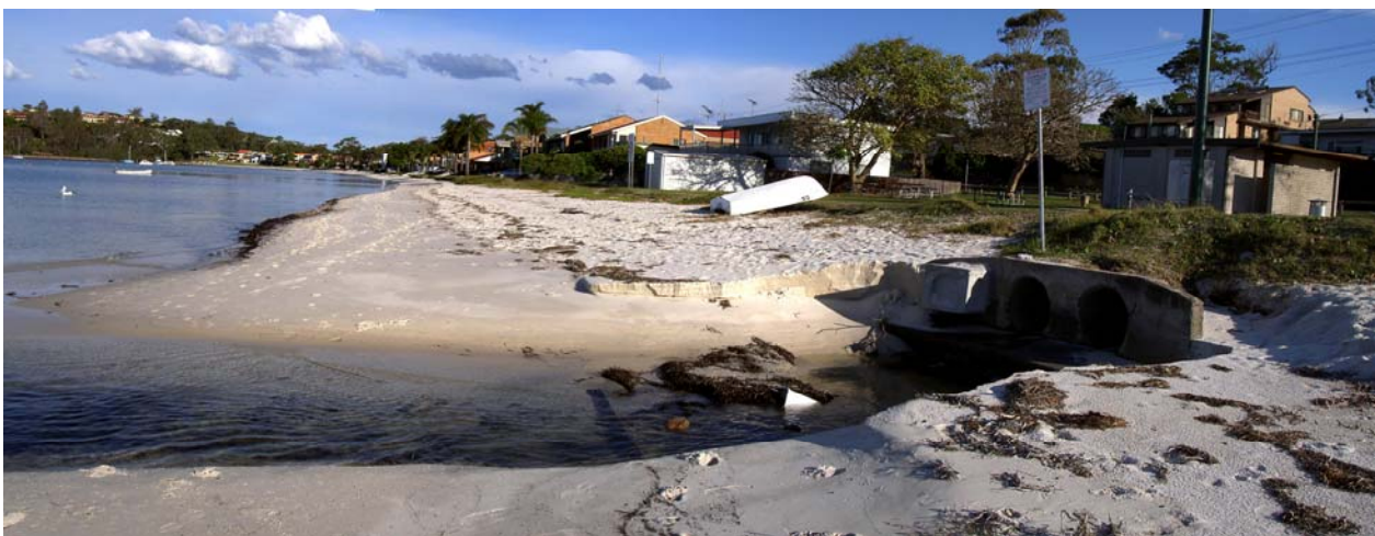
(2) Stormwater outlet on the beach.
