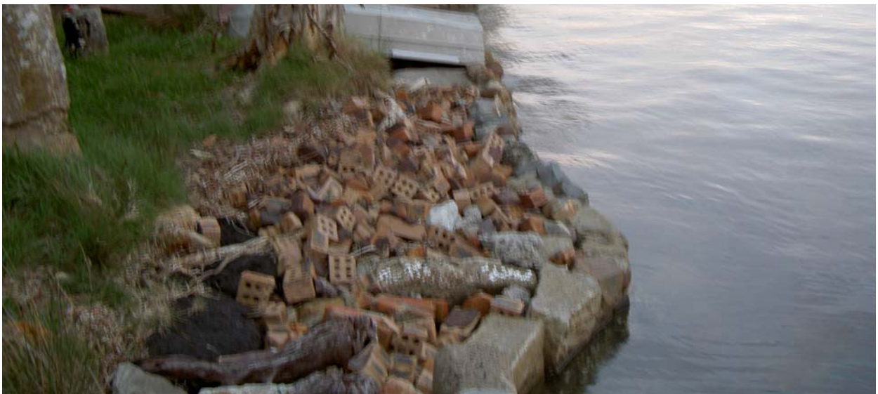
(3) Concrete and brick-bat revetment.
