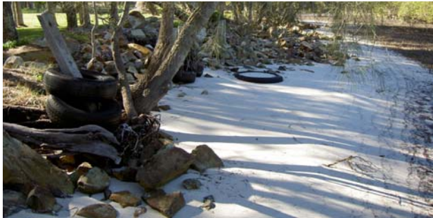
(2) Strewn rock rubble, tyre, rock and pole groyne foreshore protection structures.
