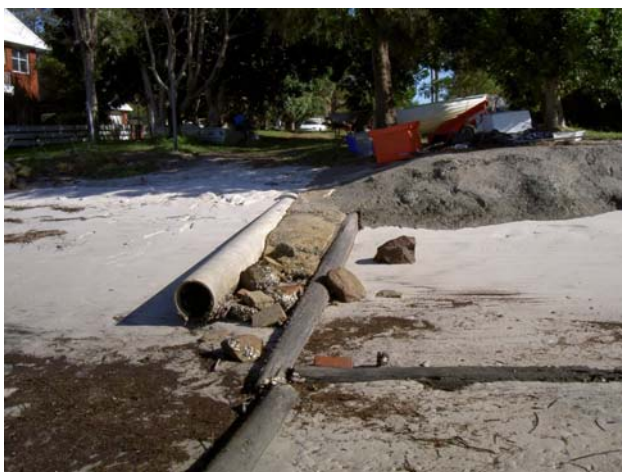
(4) Stormwater drainage across reserve.
