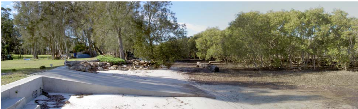
(3) Foreshore reclamation and boat ramp access flanked by rubble protection.
