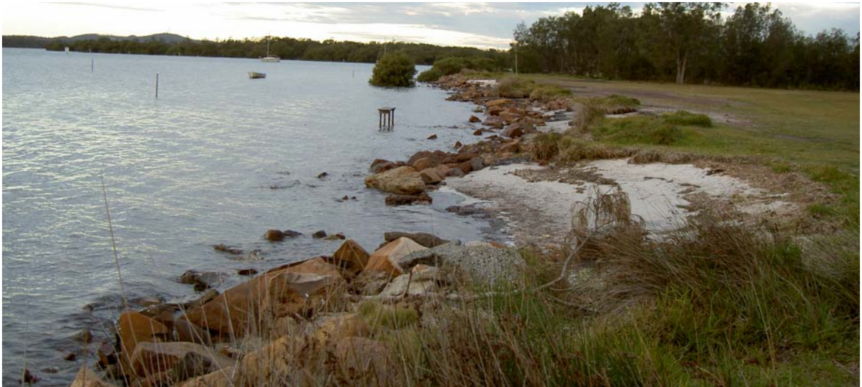
(1) Dumped rock rubble at foreshore reserve.
