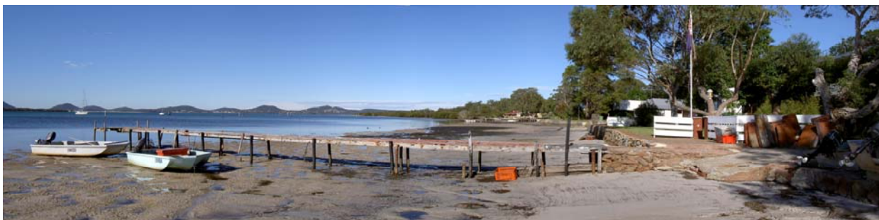
(1) Foreshore reclamation, sea wall protection and Jetty.
