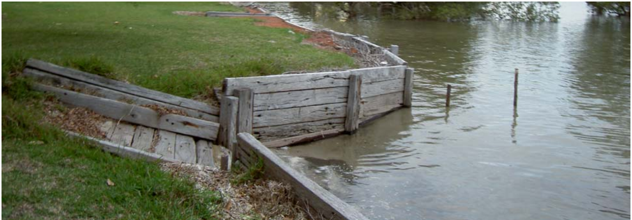
(1) Timber revetment and boat-launching ramp.
