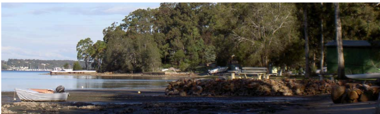
(4) Typical reclamation with rock rubble protection – south end.
