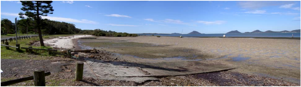
(1) Boat ramp looking east.
