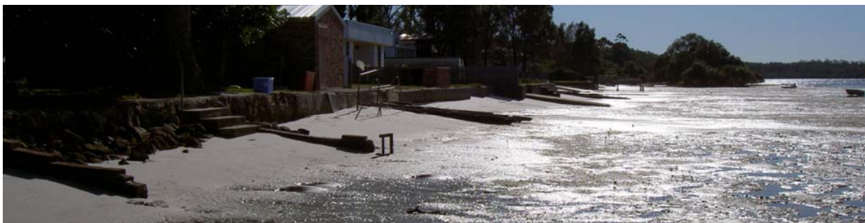
(3) Foreshore reclamation, seawall and groyne protection.
