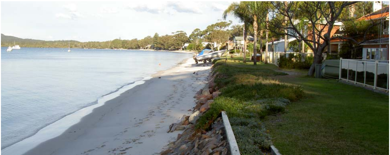
(2) Northern residences with rock protection works
