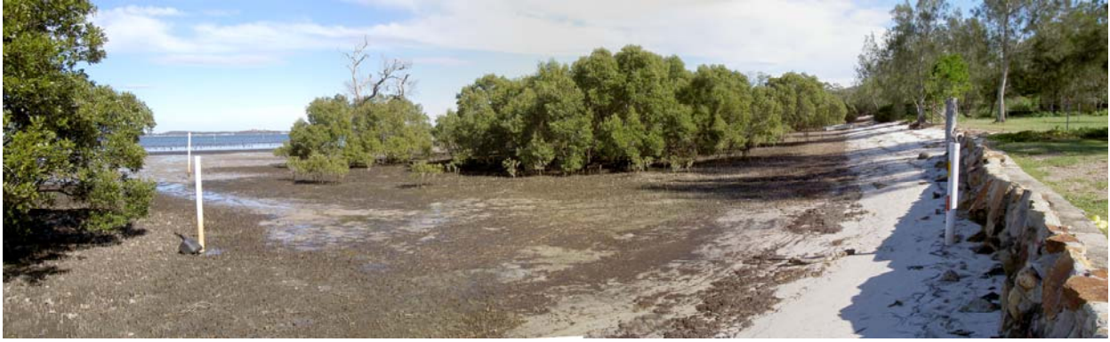
(1) Foreshore protection at boat access way through mangroves.
