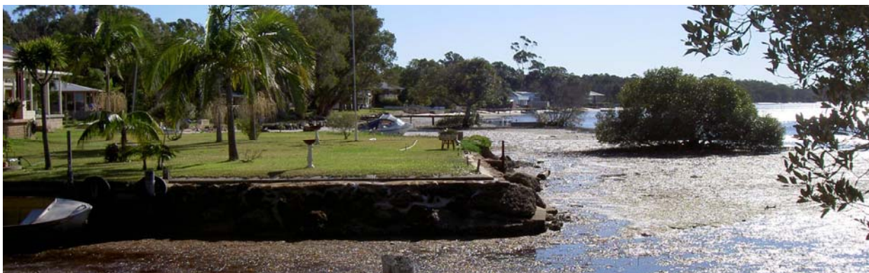
(2) Foreshore reclamation and seawall protection.
