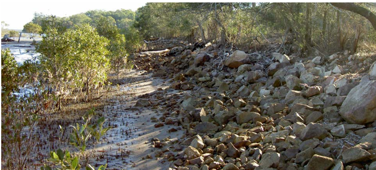
(2) Dumped rock rubble.
