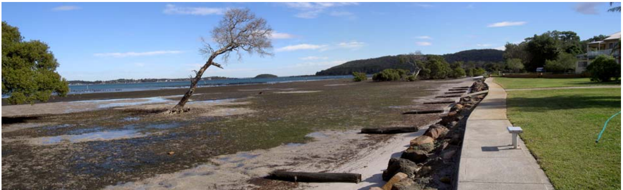
(3) Foreshore reclamation, masonry sea wall and log groynes.
