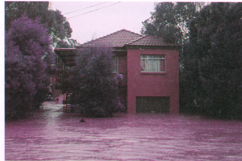
"Flood Proofing with Habitable Areas on Upper Floors" (Source: Floodplain Development Manual, pg: 50)
