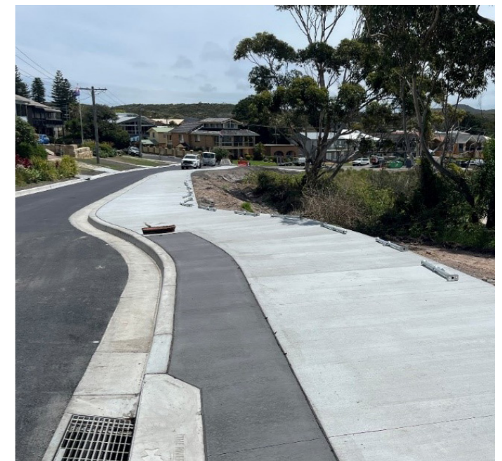
Landslip rectification works at Marine Drive, Fingal Bay
