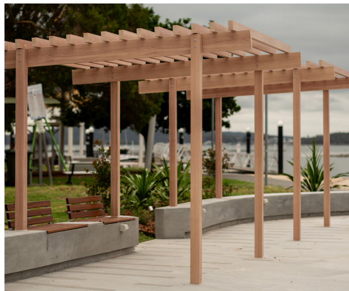
Works complete at Lemon Tree Passage Town Centre
