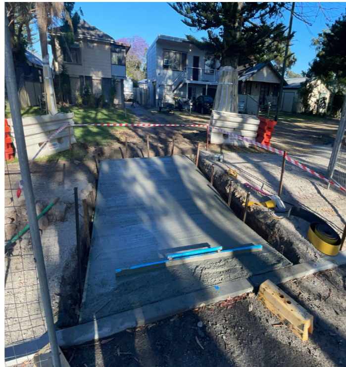
Works in progress at Avenue of the Allies, Tanilba Bay
