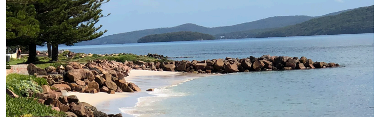
Existing groyne at Sandy Point, Corlette
