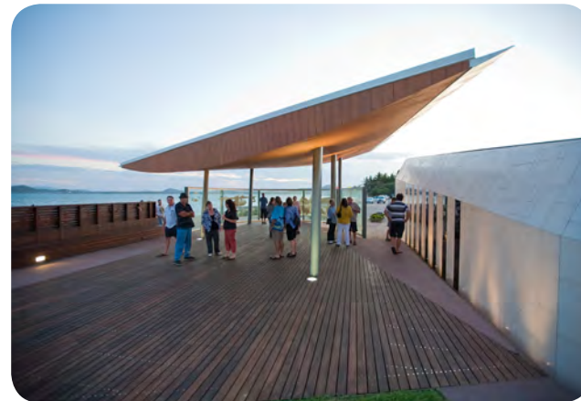
Bowen Foreshore - Boardwalk decking to stop and ponder the view Source: Tract
