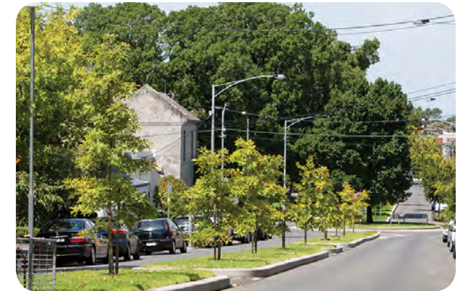
Gipps Street Upgrade - Use of Median Street Trees and focuses on drainage
