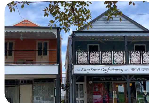
King Street Heritage Precinct
