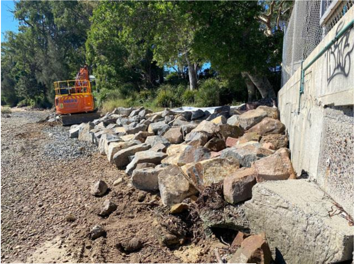
Pictured: Construction of new revetment rock wall at Soldiers Point
