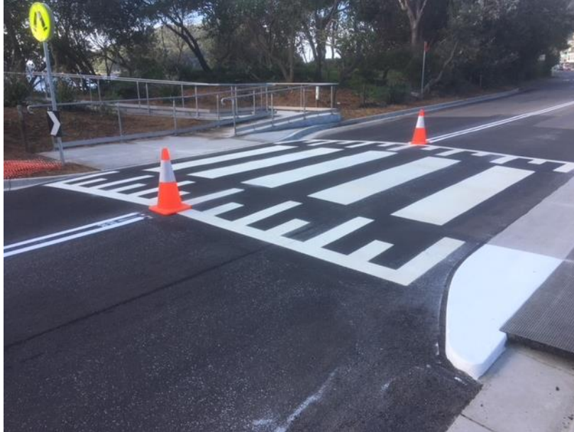
Shoal Bay safety upgrades
