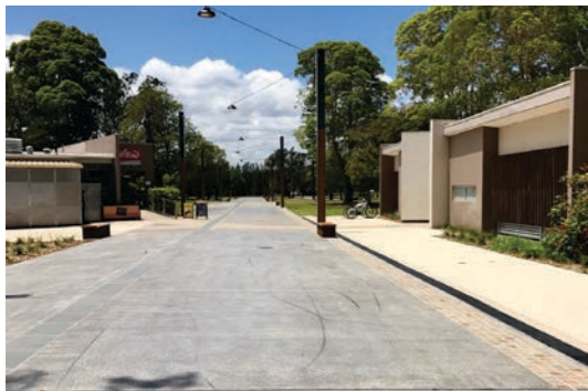
Speers Point Park, Lake Macquarie; Pedestrian spines also become service corridors for deliveries and service infrastructure.
