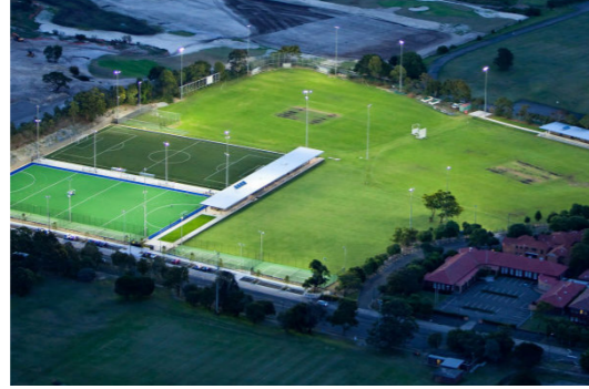
David Phillips Field, Sydney; Centralised, multi-sided pavilions that address and connect with all areas.
