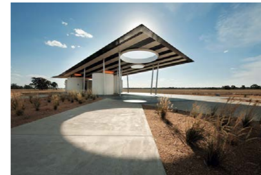
Calder Fwy Pavilion, Woodburn - BKK; Iconic architecture creates a sense of identity. Identifiable landmarks also help locate you within the Tomaree Sports Complex.
