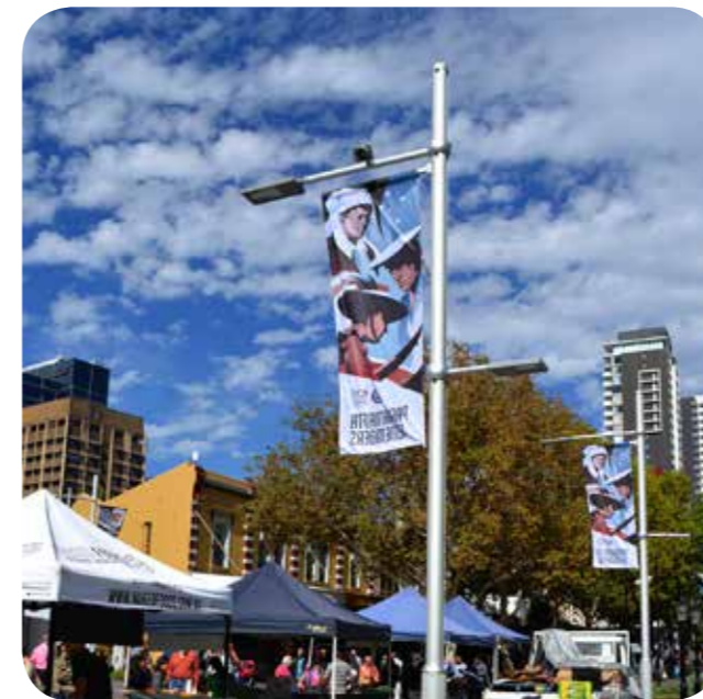
Smart Pole Lighting
