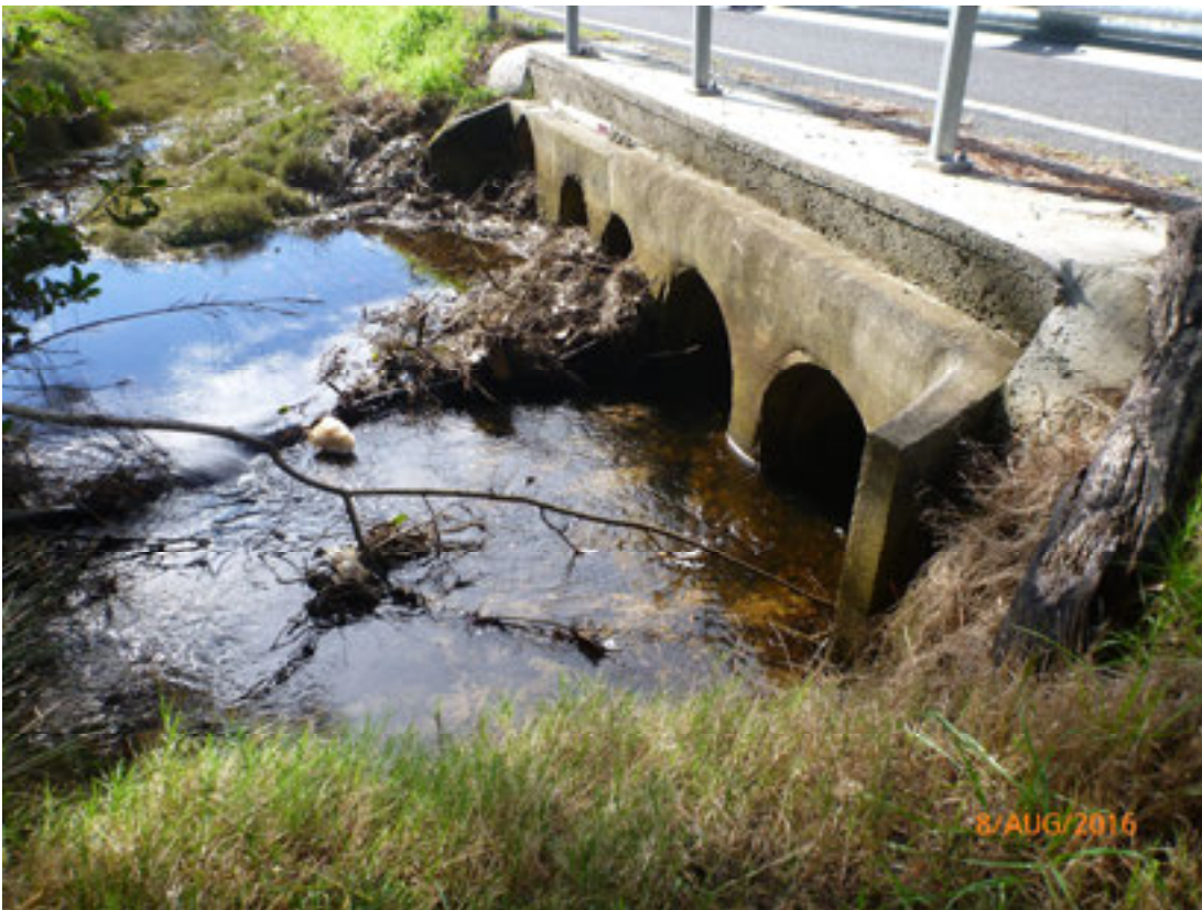
Figure 10-7 Debris accumulation propping open the same floodgate, Salt Ash
