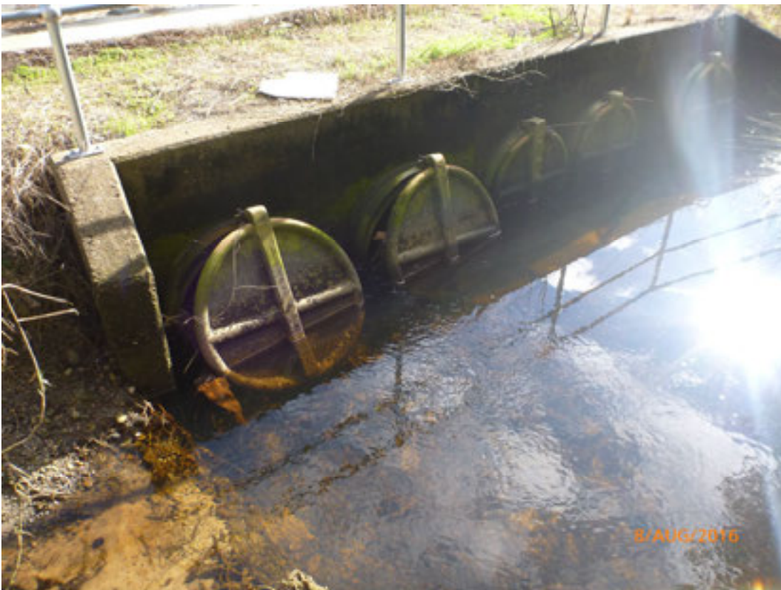
Figure 10-7 Debris accumulation propping open the same floodgate, Salt Ash
