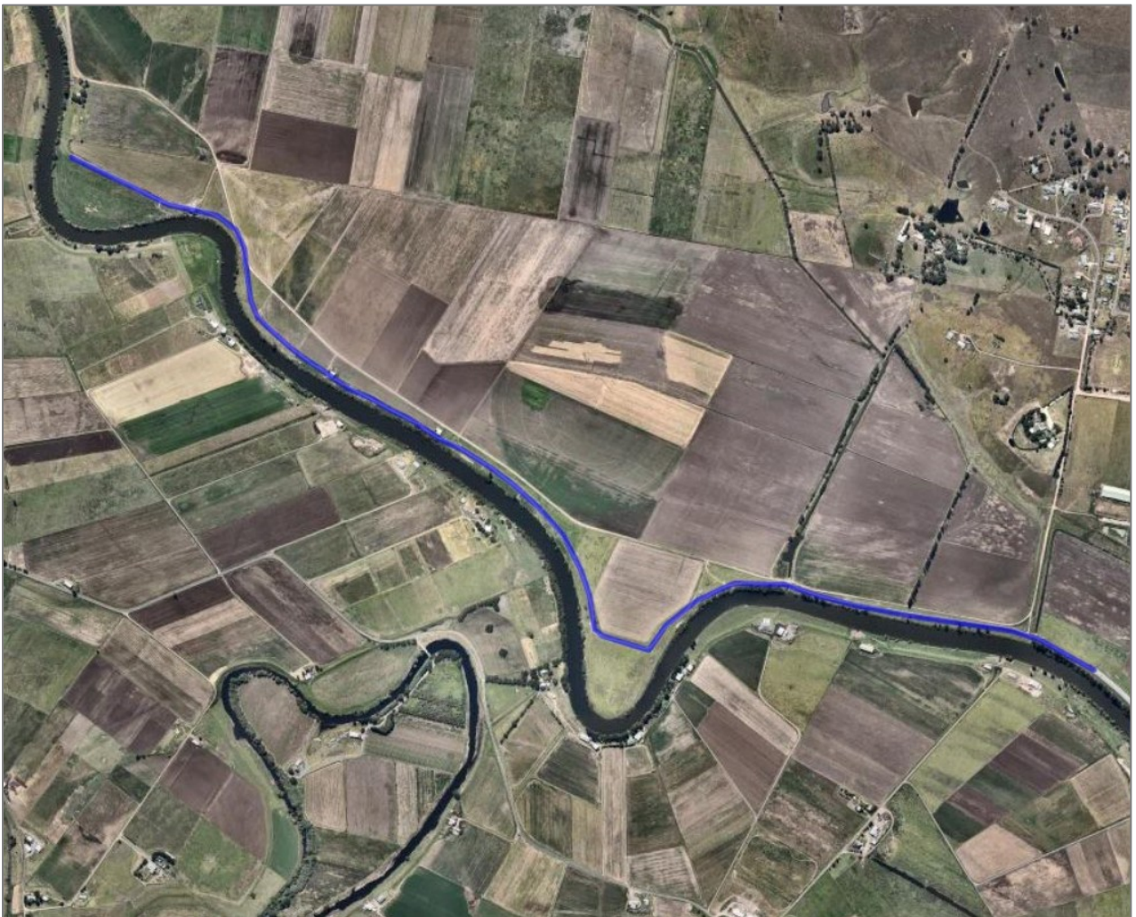
Image 1 - Extent of Levee Modification Works
