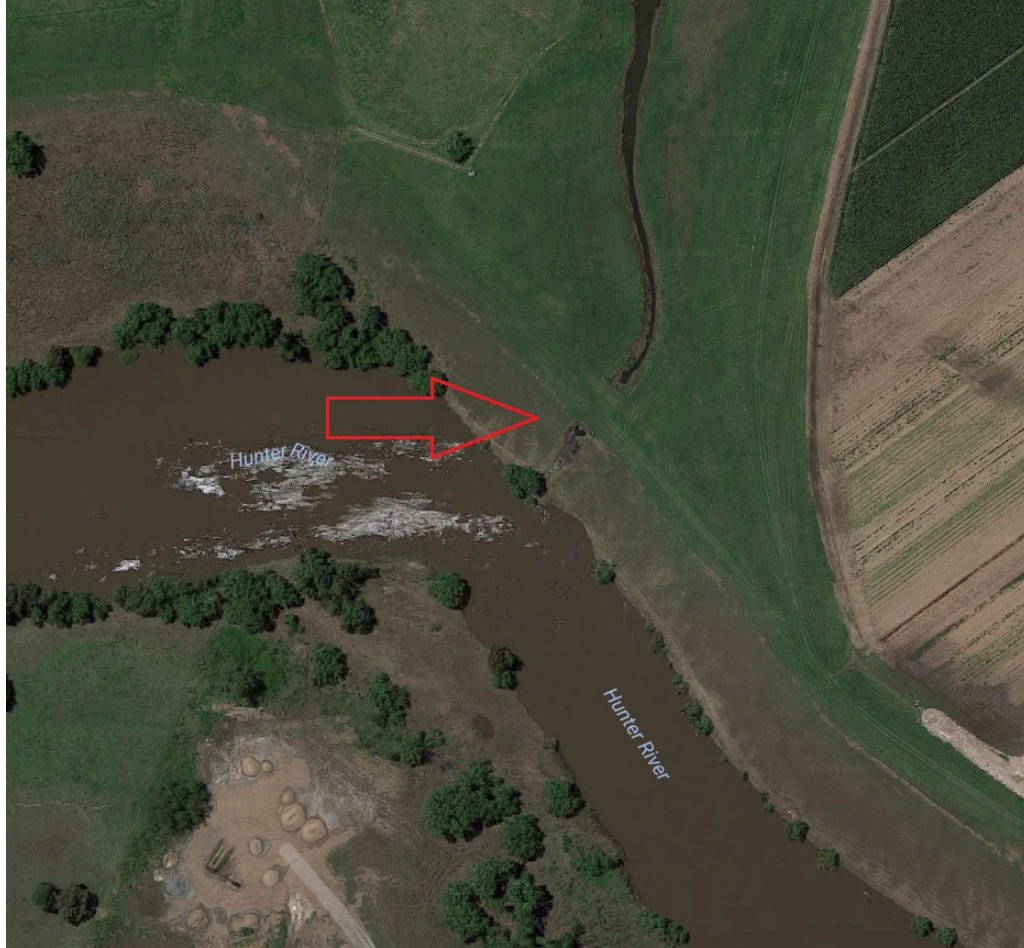
Image 3 – Narrow Gut Flood Gate
