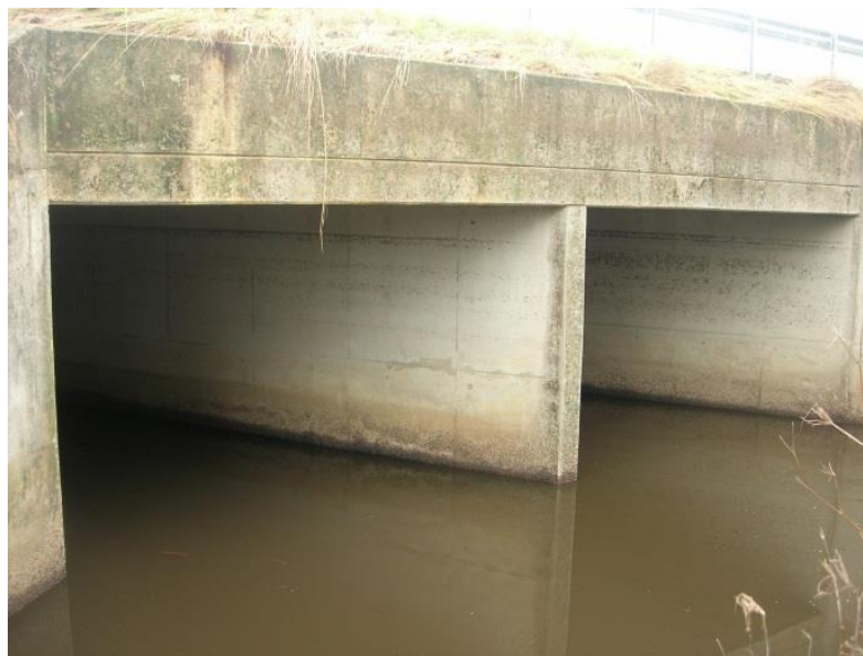
Photo 9 – Road Culverts Mindaribba
