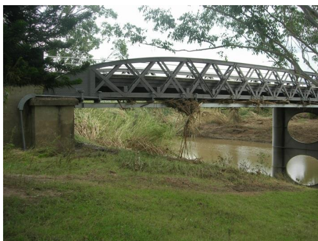
Photo 7 – Paterson Road Bridge
