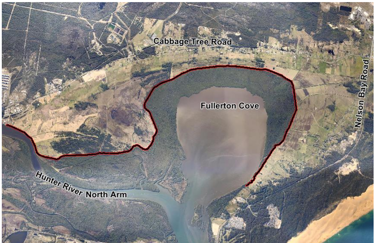
Figure 7-11 Fullerton Cove Levee
