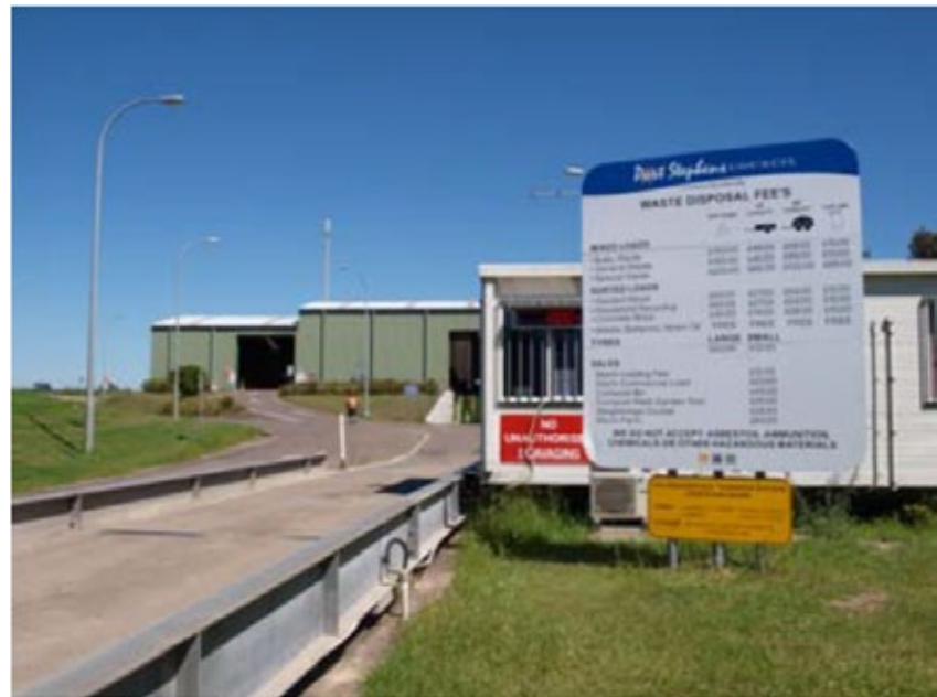
Salamander Bay Waste Transfer Station
