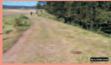
Flood mitigation levee banks
