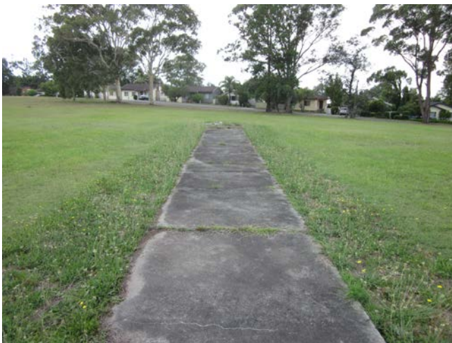
■ Plate 2: Concreted wicket on the Boomerang Park cricket pitch
