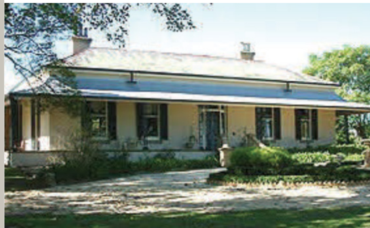
Wallalong House at Wallalong
