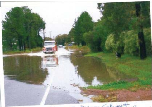
Kirrang Drive Culvert at 3 Kirrang Drive gate 2007
