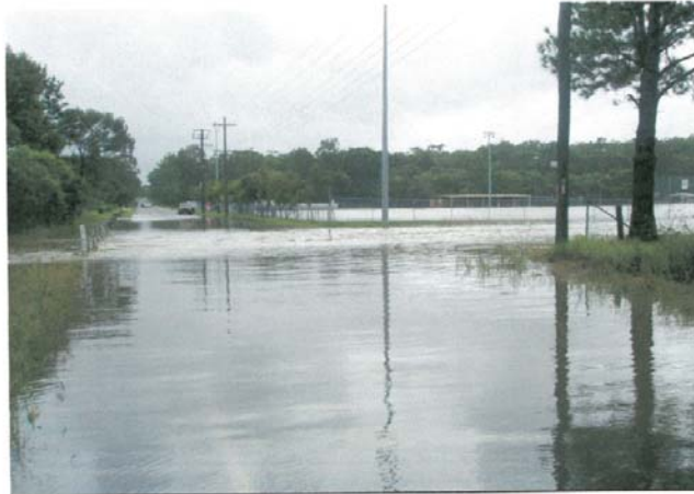
Photo taken in April 2008 following storm event. Water over Kirrang Drive level marker visible on edge of bridge
