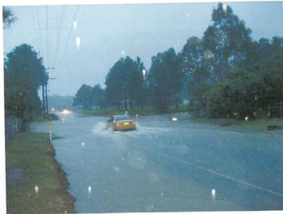
June 2007 Storm event Water over road in Kirrang Dr Campvale Drain
