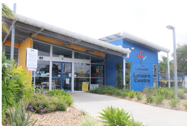
Photo: Lakeside Leisure Centre, Raymond Terrace
