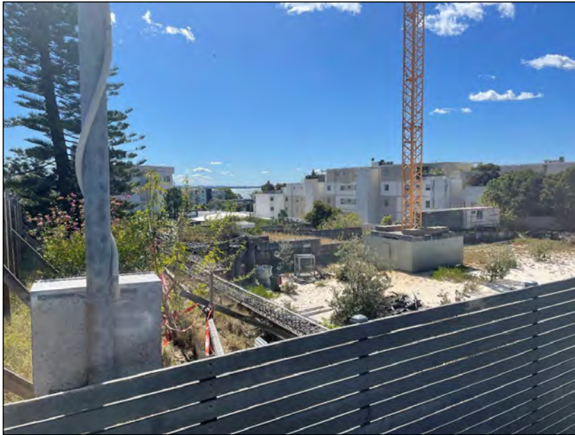
Image 5: Existing works on site.
