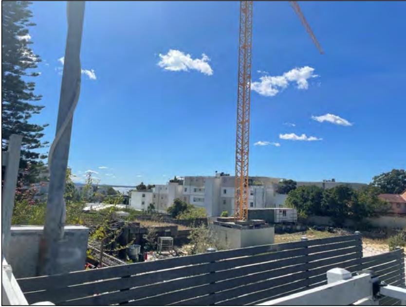
Image 3: View into site where crane and partially constructed footings exist.
