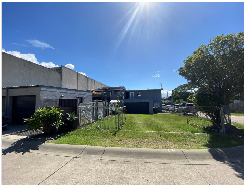
Figure 6. Rear of the site viewed from the laneway
