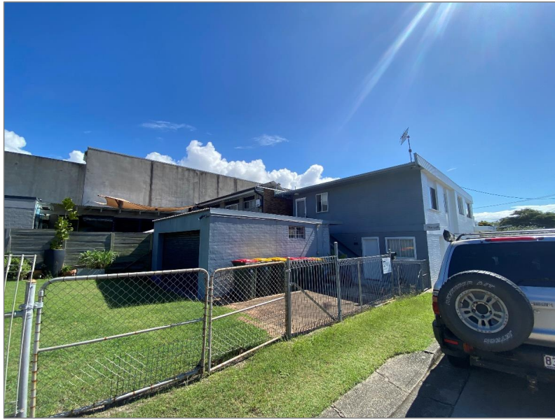
Figure 5. Rear of the existing building
