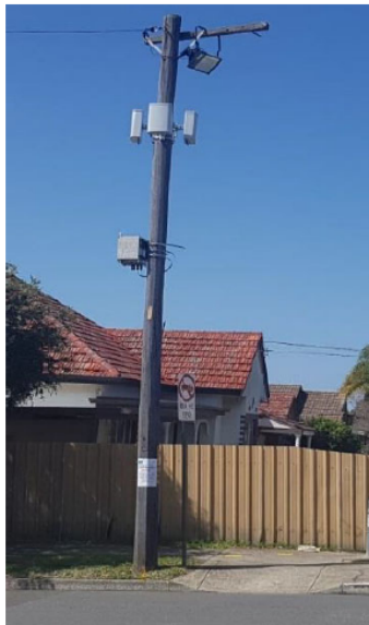
Figure 2: 5G small cell infrastructure in Canterbury on the left, older generation facilities on an existing tower in Raymond Terrace on the right.
