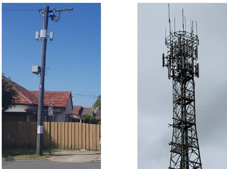
Figure 2: 5G small cell infrastructure in Canterbury on the left, older generation facilities on an existing tower in Raymond Terrace on the right.
