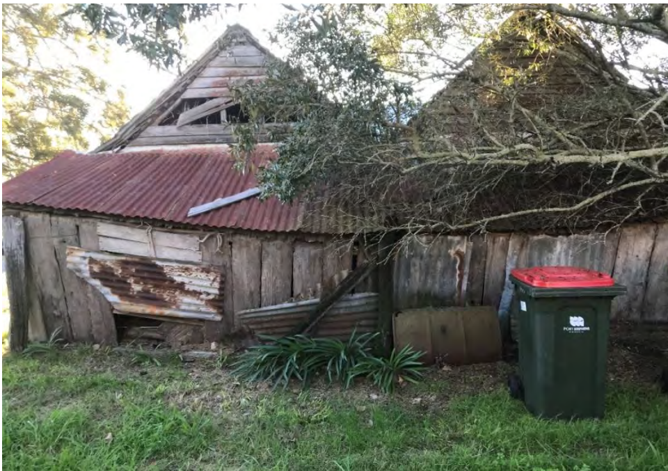
Photo 2: View of cottage looking west
