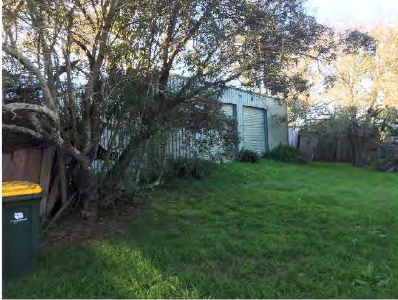
Photo 3: View of Colorbond Shed to be removed
