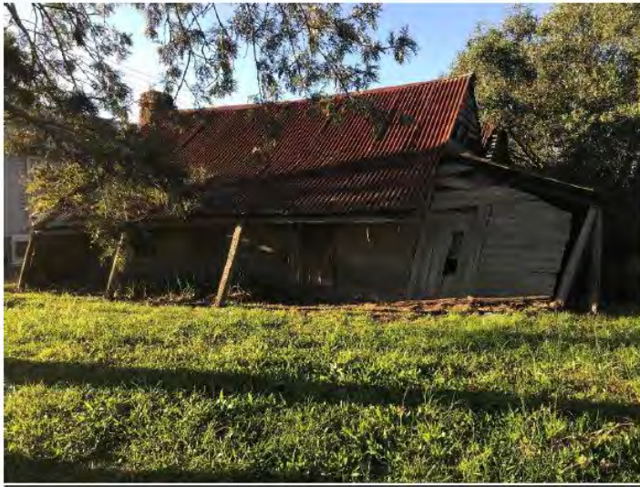
Photo 1: View of Cottage from Clarence Town Road
