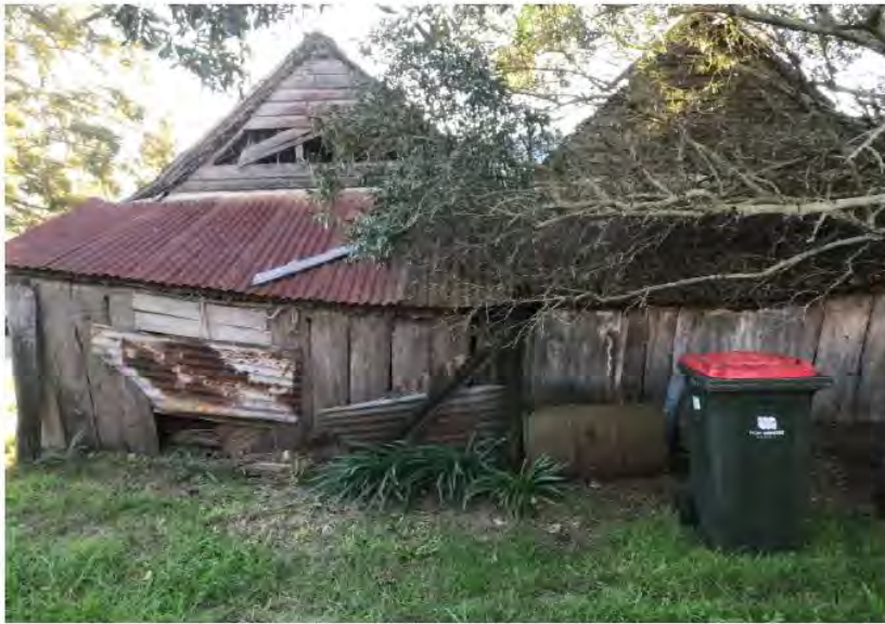
Photo 2: View of cottage looking west
