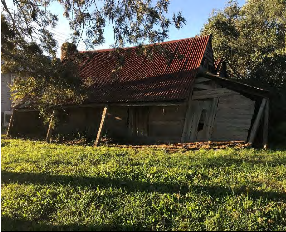
Photo 1: View of cottage from Clarence Town Road
