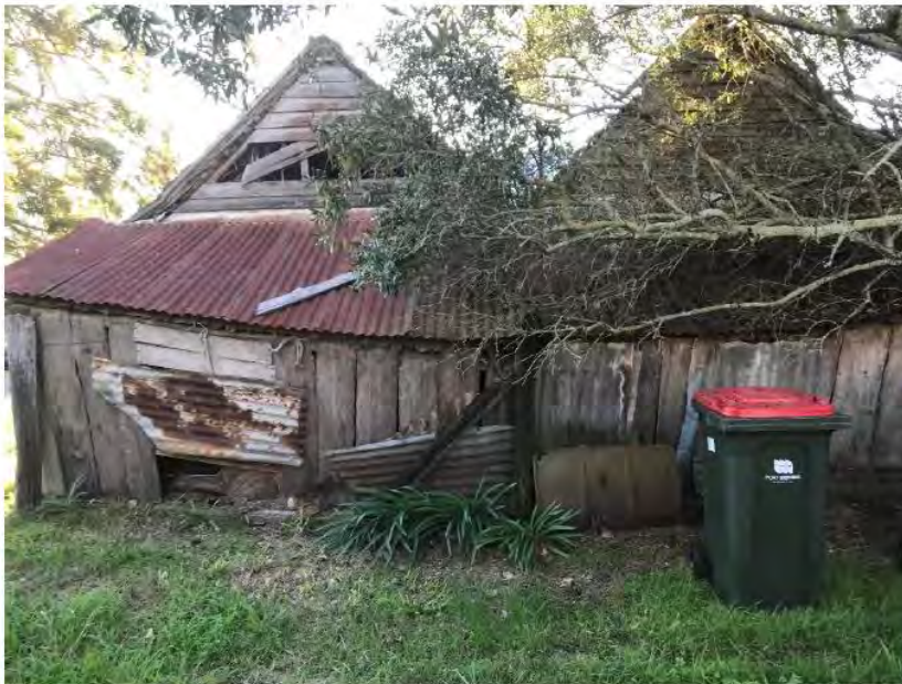
Photo 4: View of Cottage looking West
