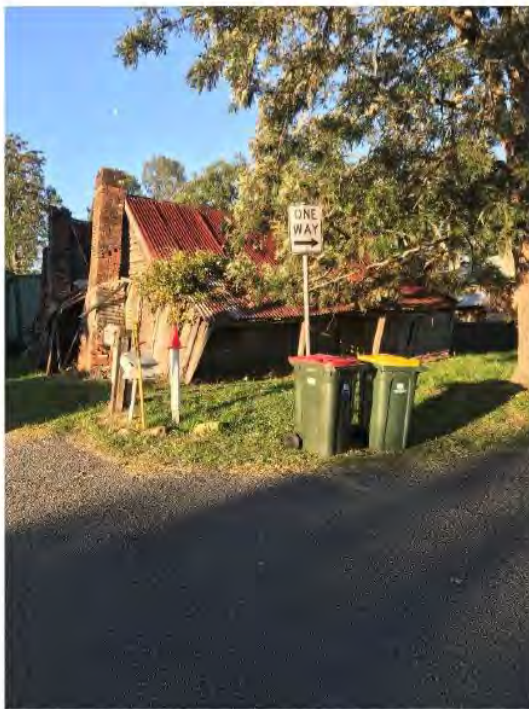
Photo 2: View of Cottage from Clarence Town Road
