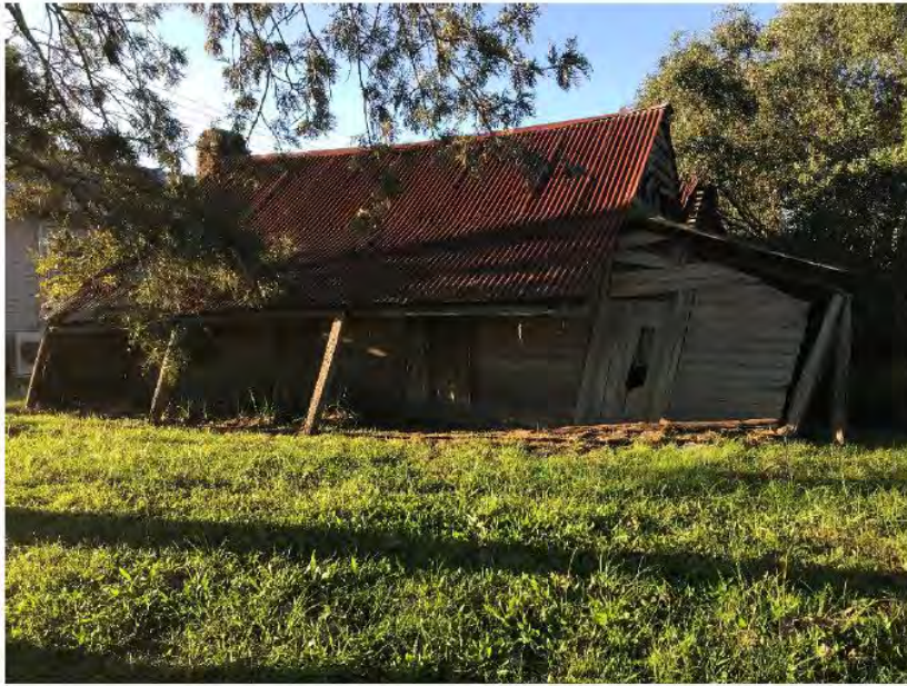
Photo 1: View of cottage from Clarence Town Road
