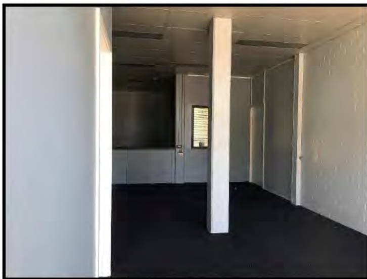
Figure 3 – Subject site, reception area, walls to be erected in background.
