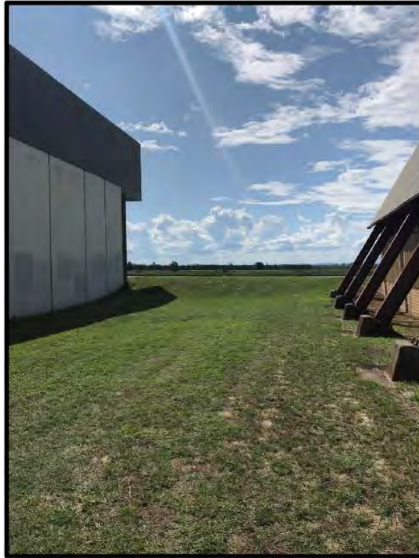
Photo 3: Subject site facing toward to the rear
