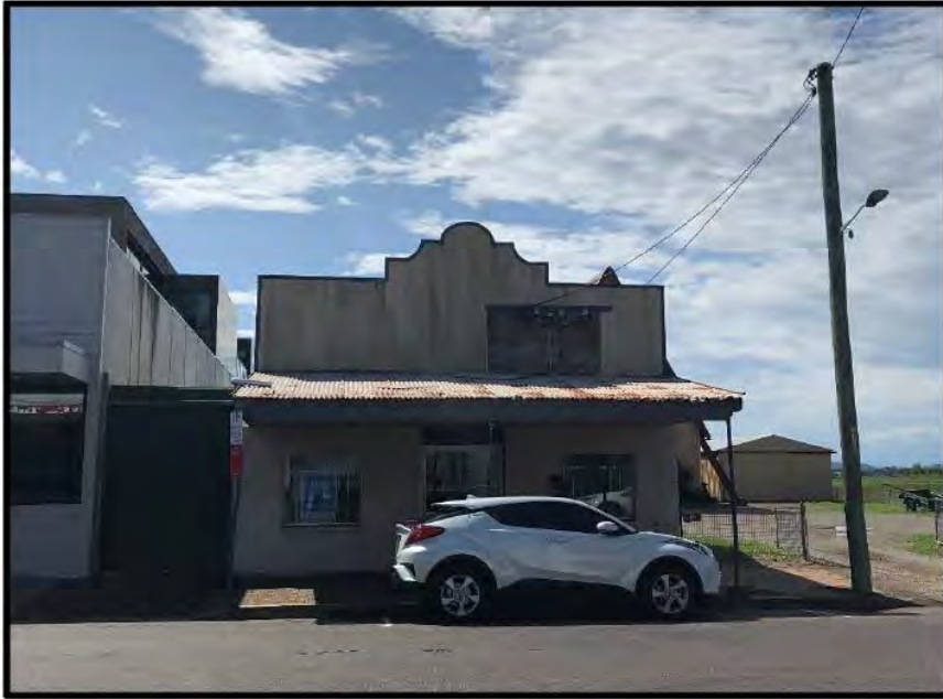
Photo 1: Existing single storey vacant building on the site
