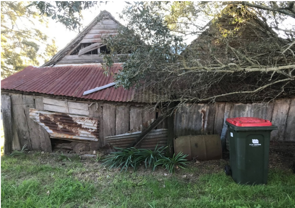
Photo 2: View of cottage looking west
