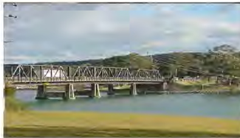
Figure 7: Karuah Bridge (Community Settlement and Infrastructure Strategy 2007)
