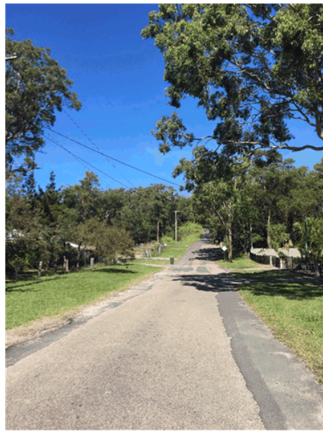
Image 3: Existing condition of Clark Street looking towards Gan Gan Road.
