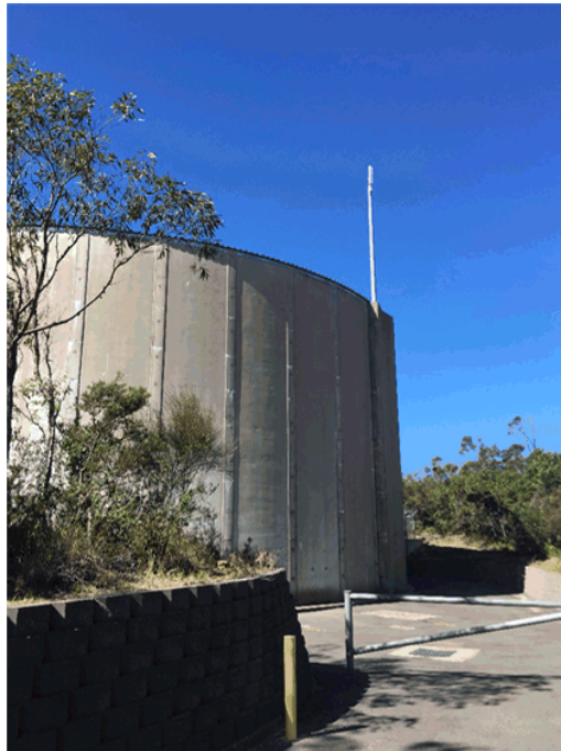
Image 5: Water reservoir and existing Freeview tower on subject site.
