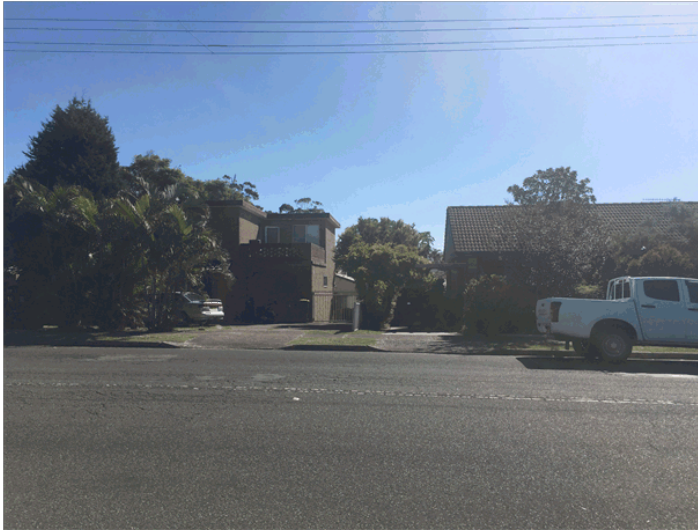
Figure 6: subject site and adjoining property to the north viewed from the eastern side of Church Street.
