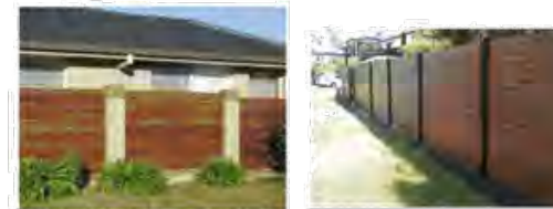
Timber panel infill atop masonry walls with masonry posts, Eastern and northern boundary. Outside sewer easement. Timber panel infill. Within easement and between properties.
