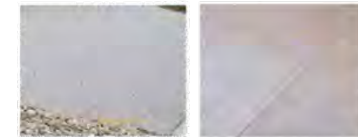
Exposed aggregate to break up the surface and define entries to buildings. Coloured concrete to driveway.
