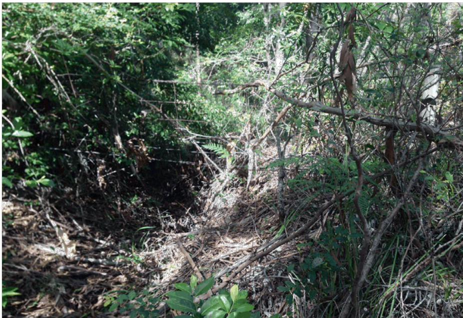
Figure 5 – Part of the proposed work area adjacent to the suspected entry to the bunker with evidence of a partial collapse
