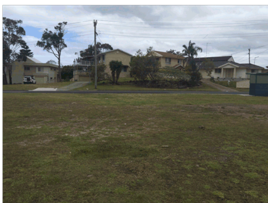
Figure 5 – View of the adjoining development to the south of the site at 1, 3 & 3A Bagnall Avenue, and 126 Soldiers Point Road
