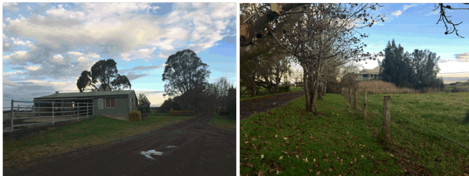
Img.1-2: Site photos: Existing structures (shed, access and dwelling)
