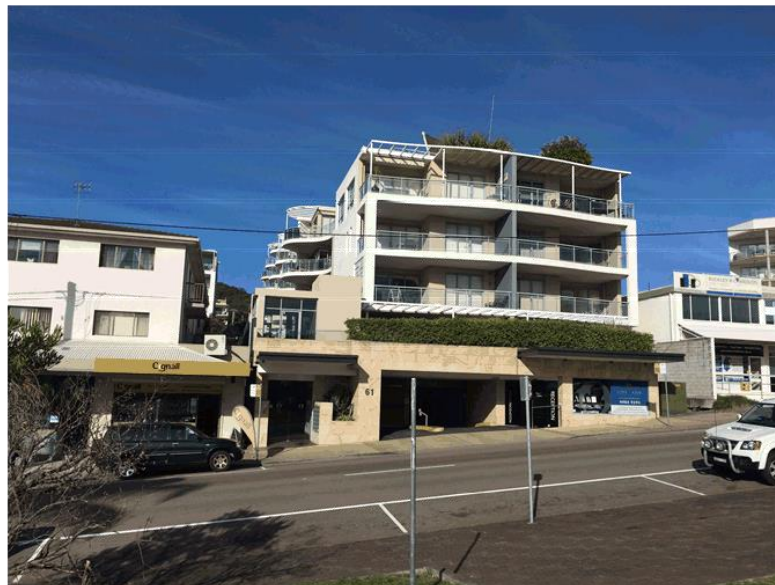
Figure 9: RFB located on 61 Donald Street.
