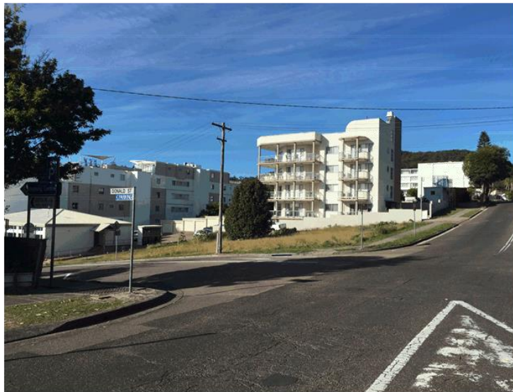
Figure 6: Facing south towards the subject site.
