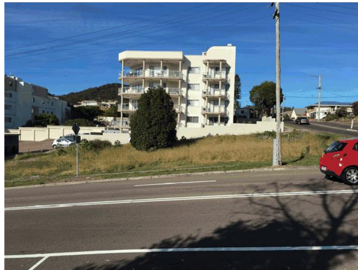
Figure 7: Illustrating the subject site south from Donald Street.
