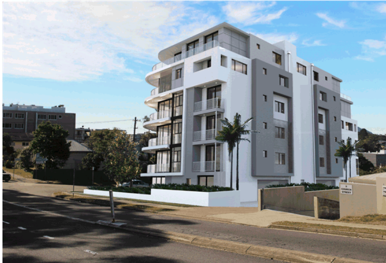
Figure 13: The southern elevation illustrating the ROW and design measures to mitigate potential privacy concerns to 9 Church Street.
