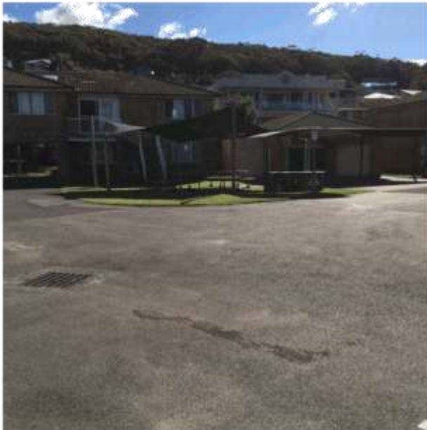
Figure 5 – existing BBQ and hardstand area between blocks B, E and managers residence
