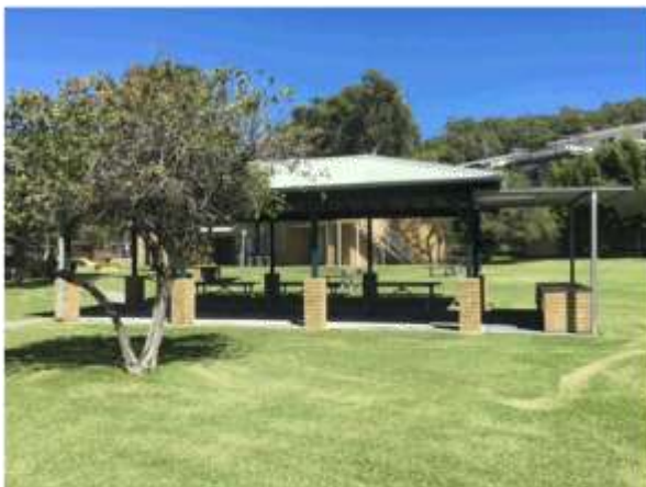
Figure 3 – Existing BBQ area
