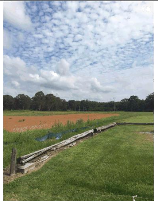
The fill placed on No. 36A under DA 16-2000-1559-1.
