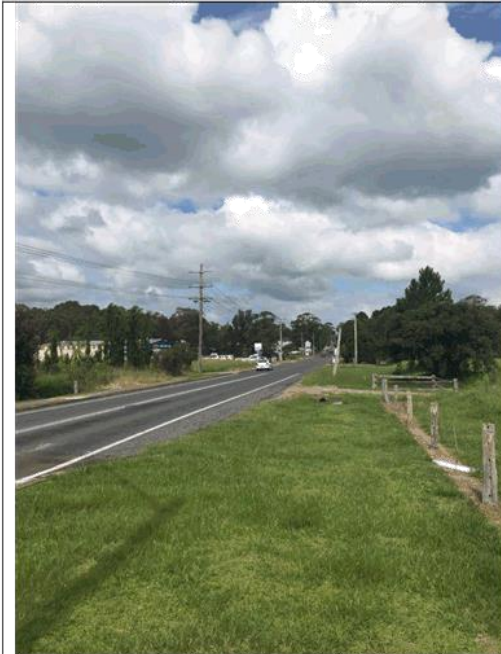
Looking east along Ferodale Road from the site frontage.
