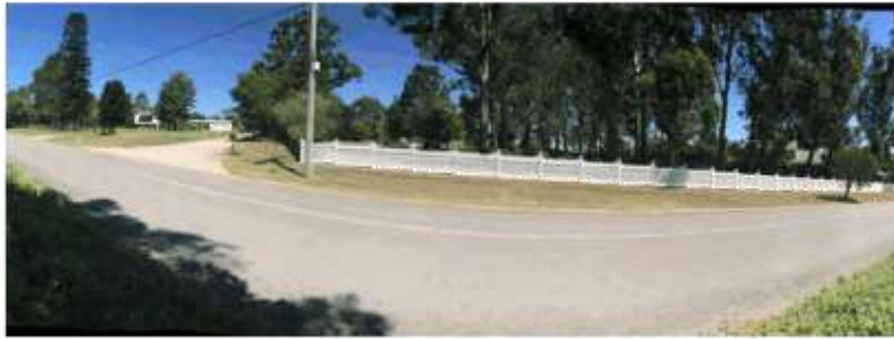
Photo 1 – View of entrance to #382 Hinton Road
