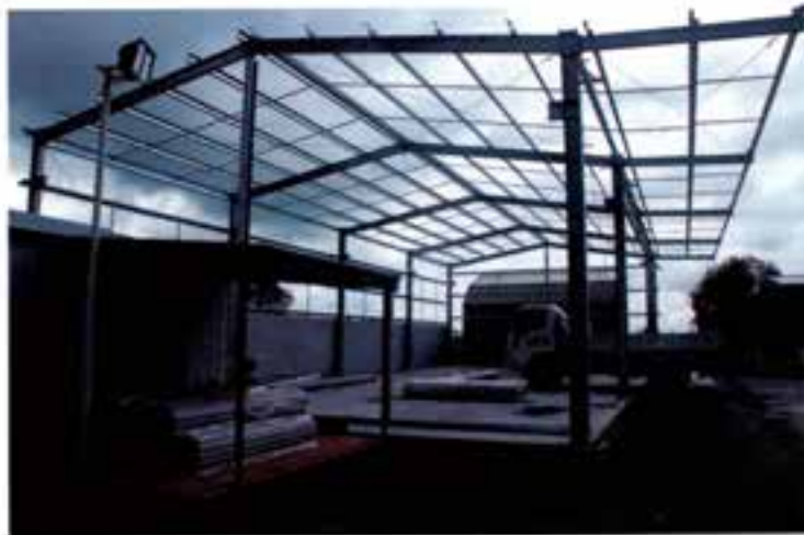
Photo 2 – Close-up view of the partially constructed shed.
