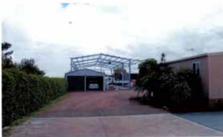
Photo 1 – The steel framework of the partially constructed rural shed viewed from the rear of the existing residence.
