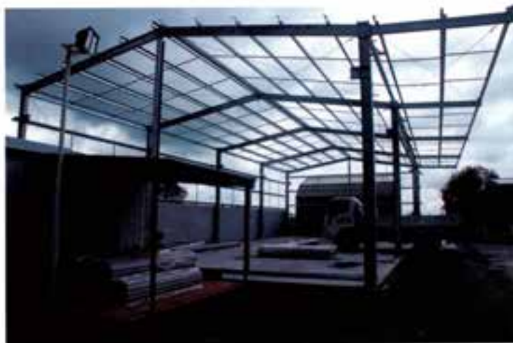
Photo 2 – Close-up view of the partially constructed shed.
